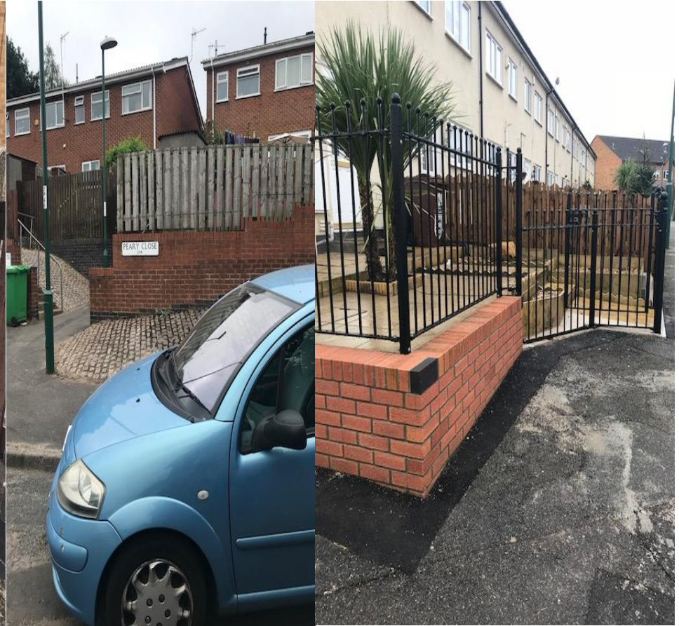
Example of new railings on brick wall
