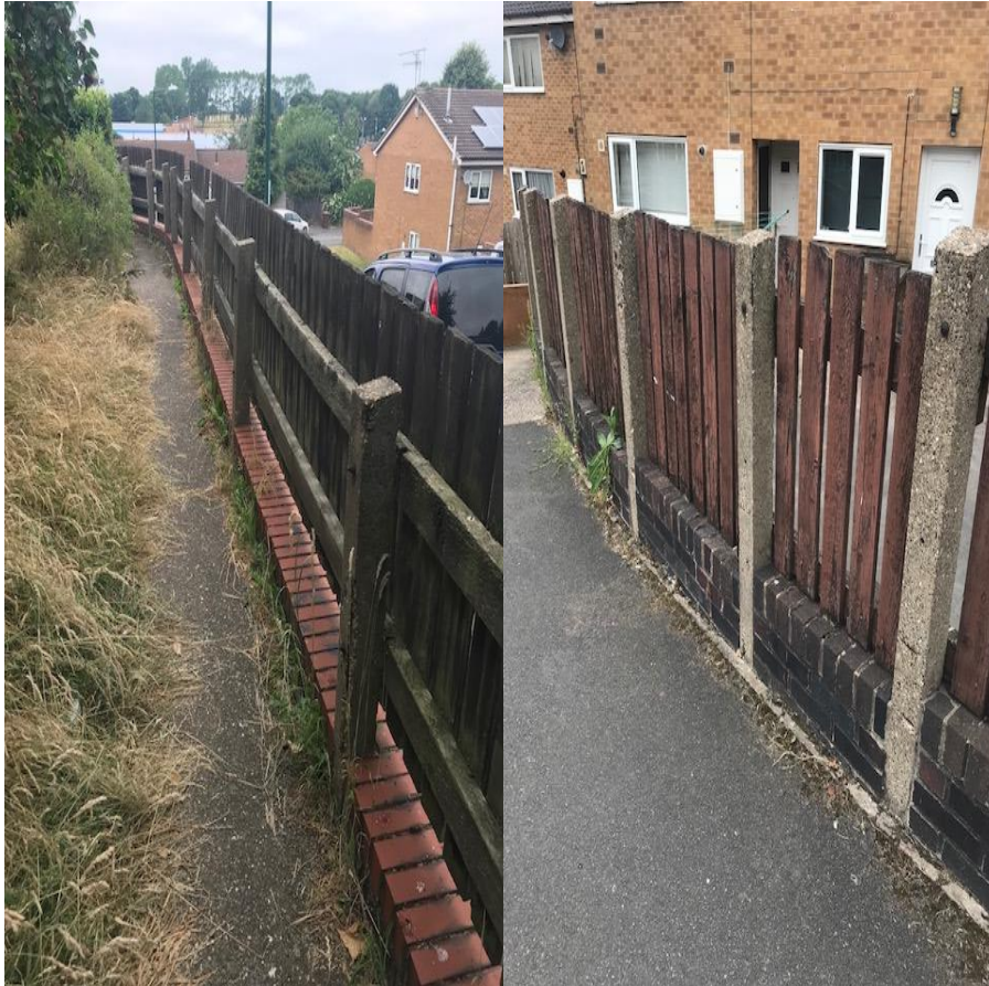
Existing timber fencing
